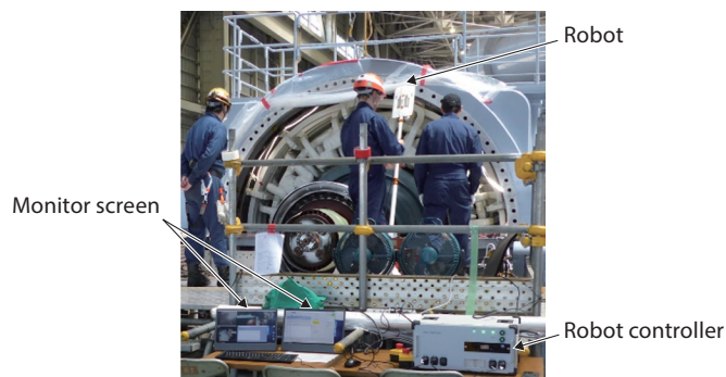
Generator inspection using inspection robot
