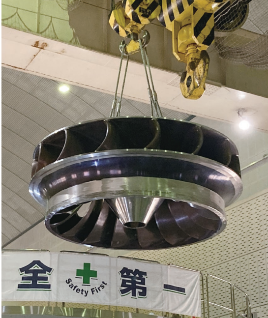
Installation of Unit 3 hydraulic runner at Okutadami Power Station
