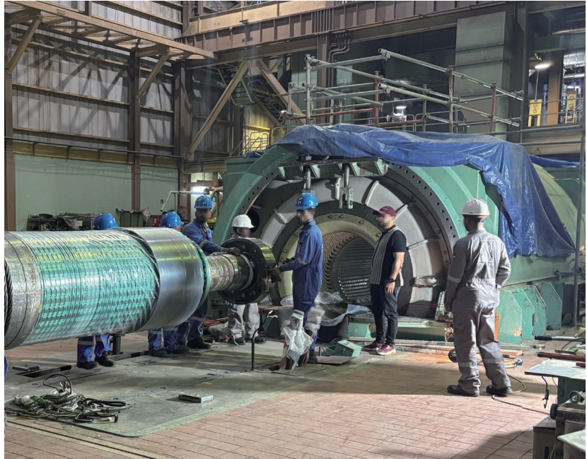
Doha East Power Plant restoration work (generator side)
