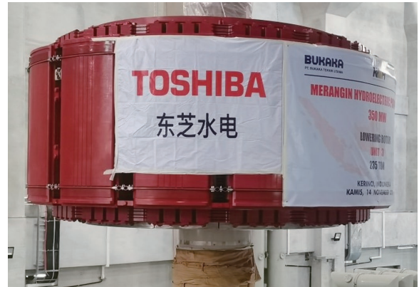
Generator rotor installation
