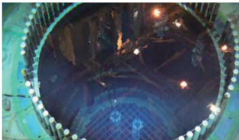
Loading nuclear fuel into reactor pool
