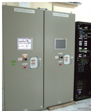
Battery control panel (front) and EMS server (back) in electric room
