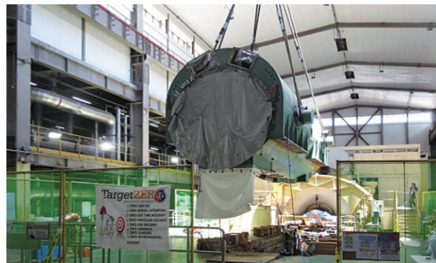
Hoisting old generator stator onto foundation after stator coil rewinding at Calaca Power Station Unit 2, Philippines
