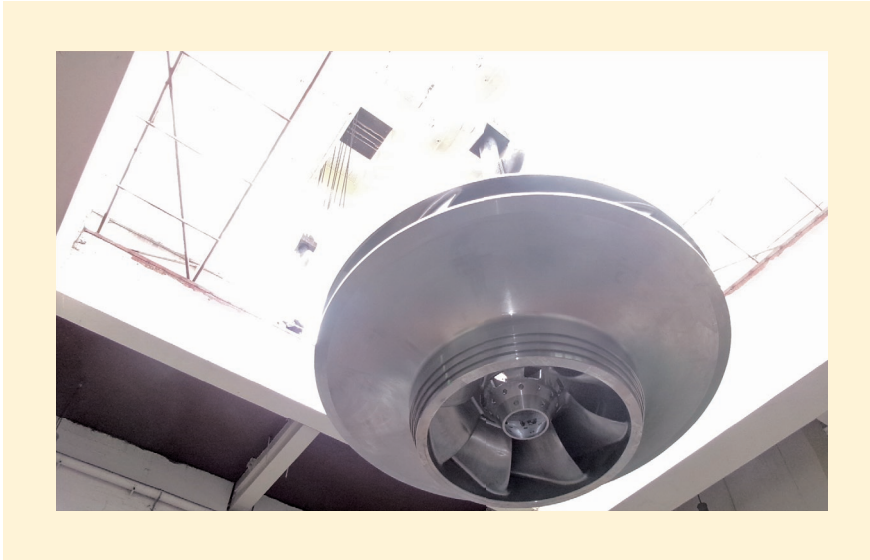
Installation of new pump-turbine runner for Unit 1 at Bajina Bašta Pumped Storage Hydropower Plant, Serbia
