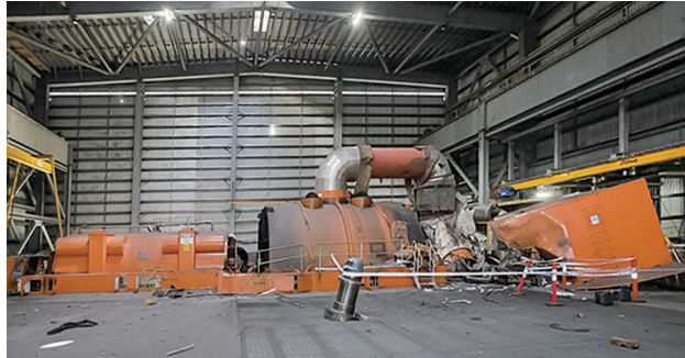
Turbine and generator at Callide Power Station Unit C4, Australia immediately after incident
