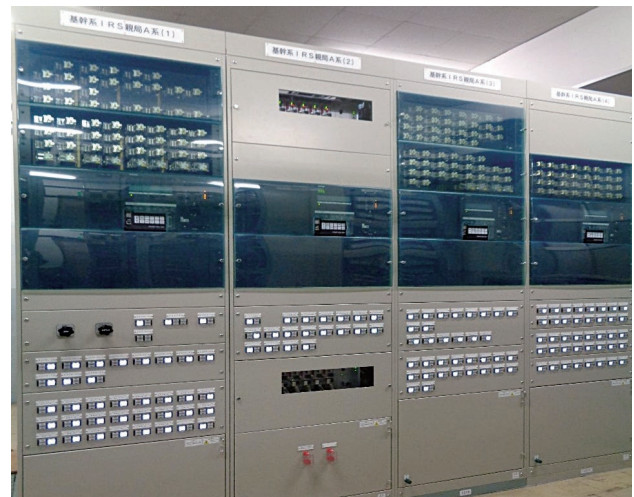
Master station (digital protective relays)
