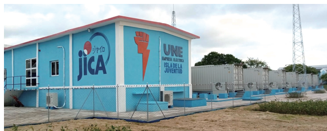
Electrical room and battery container
