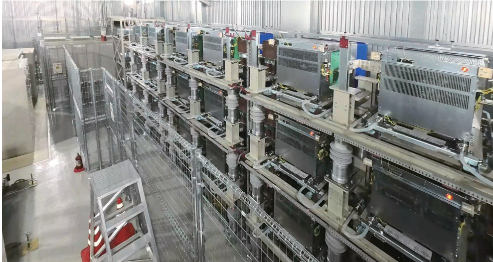
STATCOM at Shikoku Electric Power Transmission & Distribution Co., Inc. Nakamura Substation (view inside valve hall)
