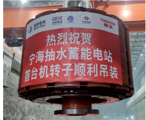
Rotor installation
