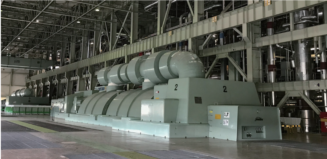
Refurbished turbine-generator equipment at Aioi Biomass Power Plant
