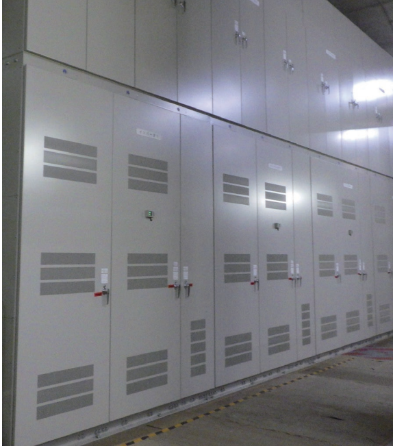
New power converter for secondary excitation device at Electric Power Development Co., Ltd. Okukiyotsu No. 2 Power Station
