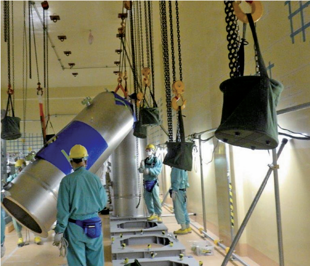
Active vessel off-gas treatment units under construction
