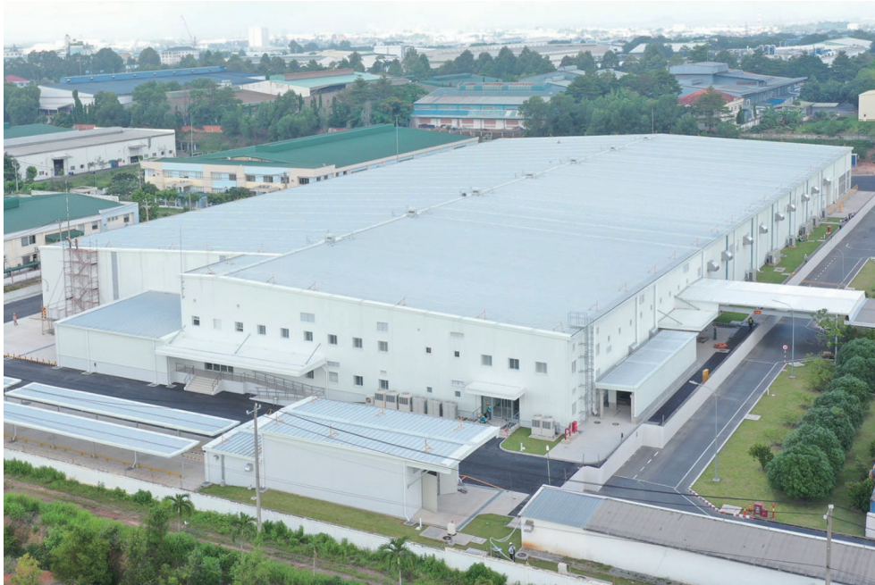
New factory in Vietnam for mass production of motors and generators for electrified vehicles
