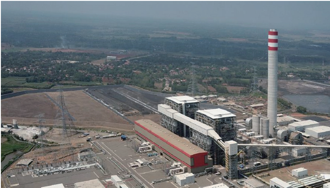
Tanjung Jati B power plant, Indonesia
