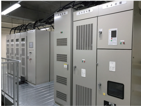
600/750 VDC TESS for railway electrification system of Hiroshima Electric Railway Co., Ltd.
