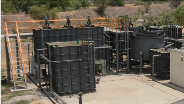
Pilot plant with upsized high-rate clarifier
