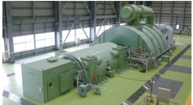
Steam turbine and generator for Noshiro Thermal Power Station Unit 3 of Tohoku Electric Power Co., Inc.
