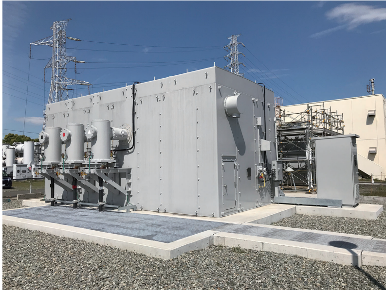
275 kV gas-insulated shunt reactor for Minami-Kawasaki Substation of TEPCO Power Grid, Inc.
