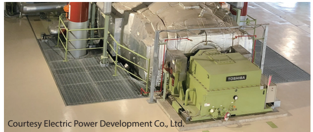
Steam turbine and generator for Takehara Thermal Power Station New Unit 1 of Electric Power Development Co., Ltd.
