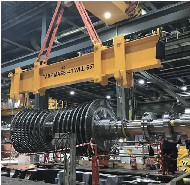
Installation of intermediate-pressure (IP) rotor at Mt Piper Power Station Unit 1, Australia
