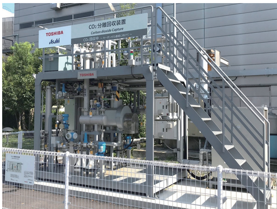
CO 2 capture test equipment at CCU facility of Asahi Quality & Innovations, Ltd.
