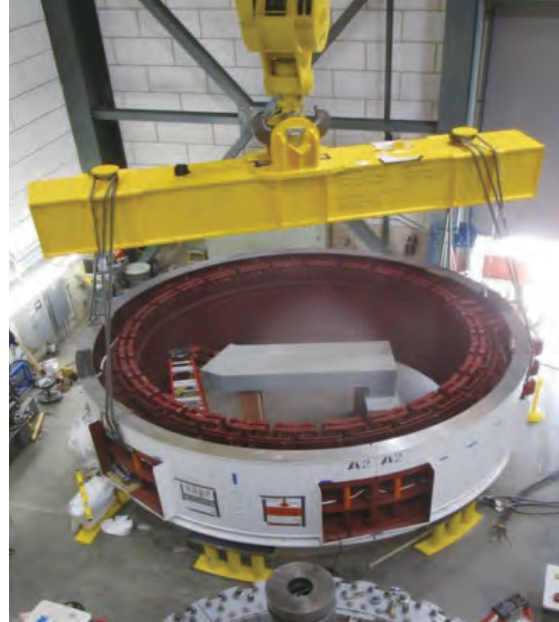
Installation of first generator stator at Blue Mesa Power Plant, U.S.A.
