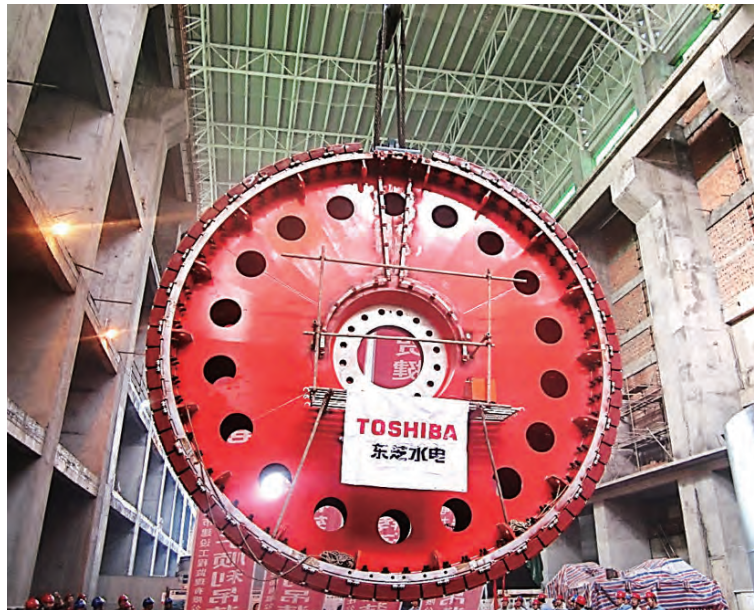
Installation of first generator rotor at Qianwei Power Station, China
