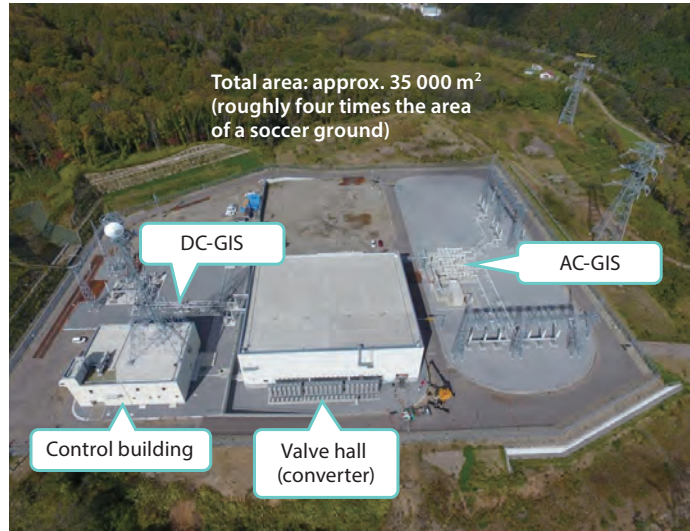
Hokuto Converter Station
