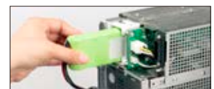
Replacement of an OS shutdown battery
