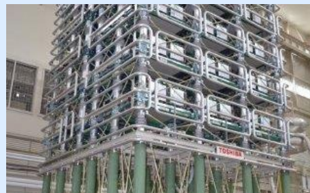
HVDC Converter (DC power transmission)
