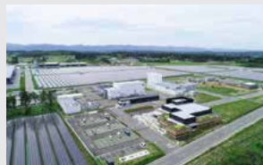
2020 World's leading scale World's leading scale H 2 energy system (Fukushima Hydrogen Energy Research Field: FH2R) * NEDO Project
