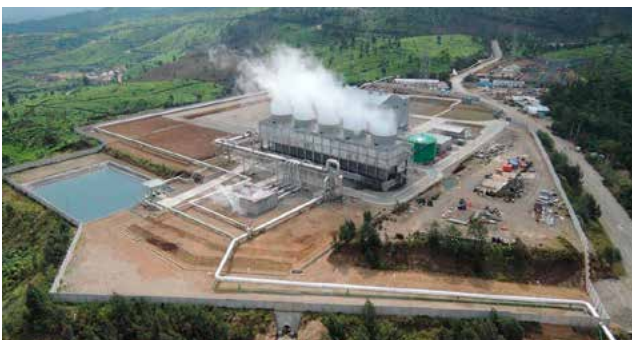
Patuha Geothermal Power Plant in Indonesia
