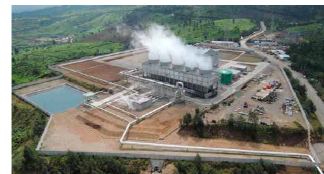
Patuha Geothermal Power Plant in Indonesia
