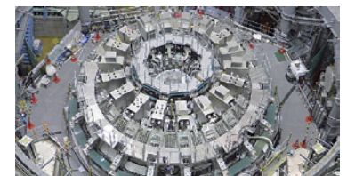
JT-60SA / 真空容器現地組立 JT-60 Super Advanced / Vacuum Vessel Installation (Courtesy of QST)
