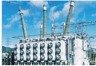
500kV-1000MVA 分解輸送型三相変圧器 (中部電力株式会社西部変電所) 500kV-1000MVA 3-Phase ASA (Advanced Site Assembly) Transformer (Seibu Substation of Chubu Electric Power Co., Inc.)
