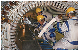
発電機補修 Electrical generator repairing
