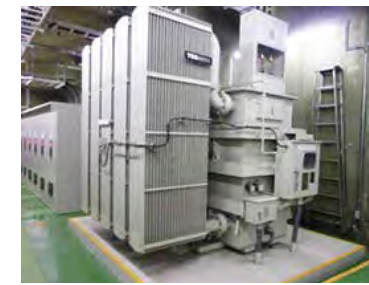
Gas Insulated Transformer
