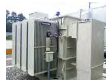
Gas Insulated Transformer
