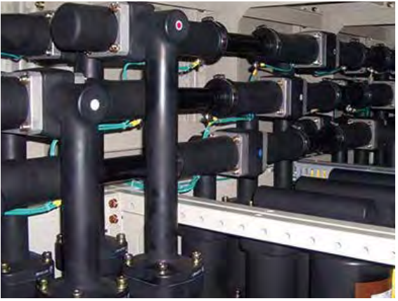
SIS Busbar Compartment
