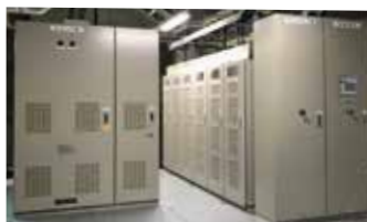
Traction energy storage system with SCiB™ for DC railway power supply systems (for Okinawa Urban Monorail, Inc.)
