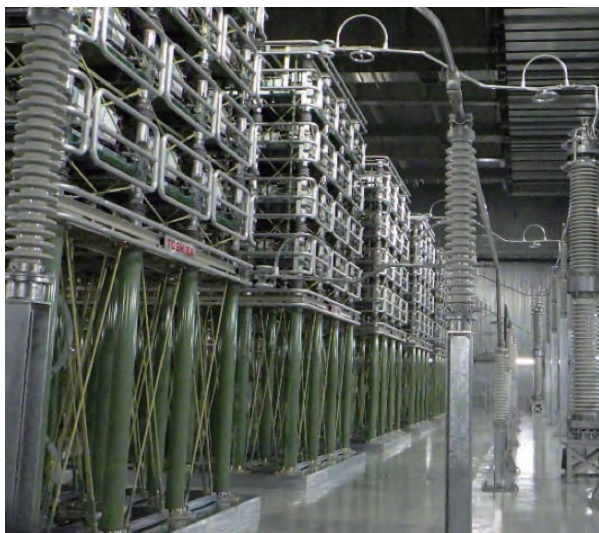
自動式変換器 Voltage source converters for New Hokkaido-Honshu High-Voltage DC (HVDC) Link
