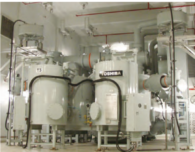
地下変電所に設置したGIT Gas-insulated transformers (GITs) installed at underground substation of Toronto Hydro-Electric System Ltd., Canada
