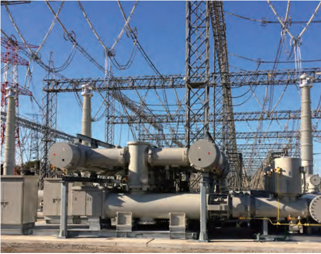
新佐原変電所に設置した550 kV GIS 550 kV GIS installed at Shin-Sawara Substation of TEPCO Power Grid, Inc.
