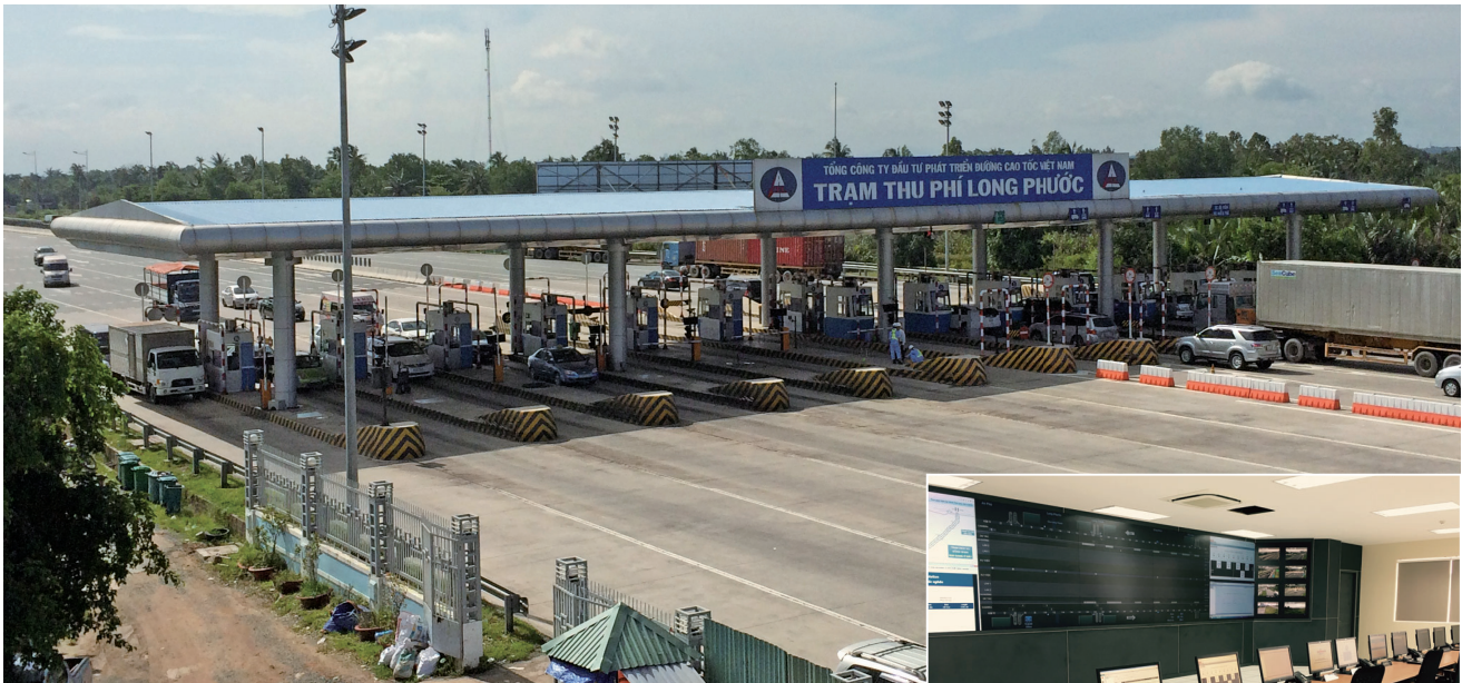
Toll gate equipped with ETC system
