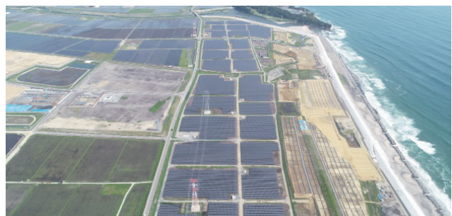
Minamisoma Haramachi-Higashi Solar Power Plant (32.3 MW DC)
