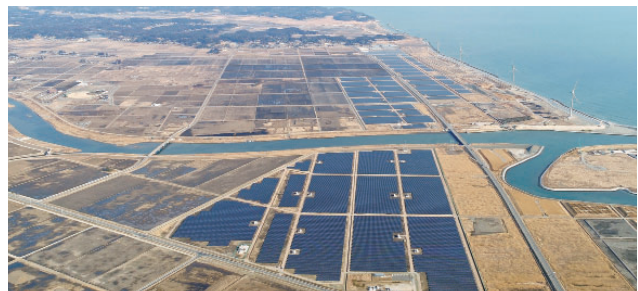
Minamisoma Mano-Migita-Ebi Solar Power Plant (59.9 MW DC)
