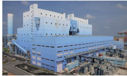
Overall view of Talin Power Plant New Units 1 and 2
