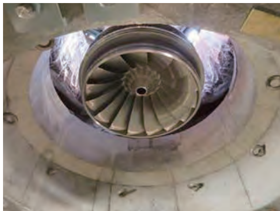
早川第三発電所2号機の水車ランナ Hydraulic runner for Hayakawa Daisan Hydroelectric Power Station Unit 2 of Tokyo Electric Power Company Holdings, Inc.
