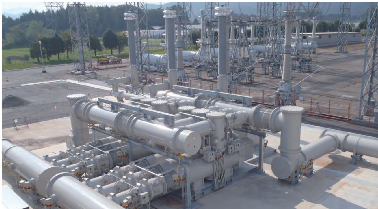
新信濃変電所 550 kV ガス絶縁開閉装置 550 kV gas-insulated switchgear for Shin-Shinano Substation of TEPCO Power Grid, Inc.
