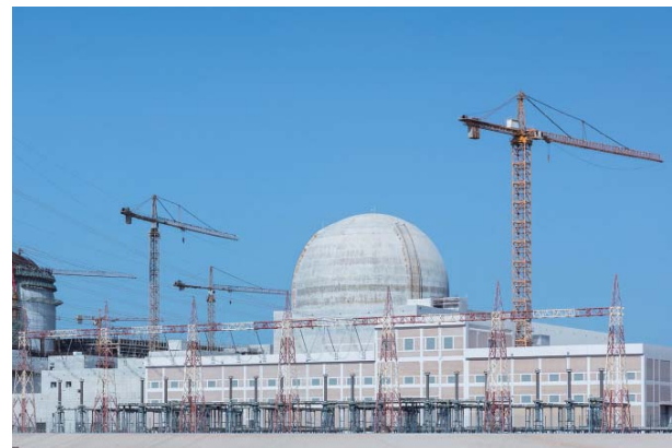
Switchyard of Barakah Nuclear Power Station Units 3 and 4, UAE
