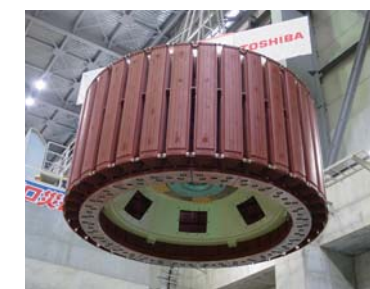
Installation of rotor in pit
