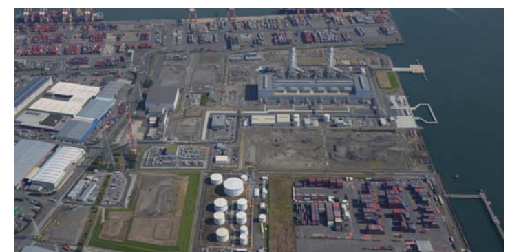
Overview of Nishi-Nagoya Thermal Power Station Unit 7-1 of Chubu Electric Power Co., Inc.
