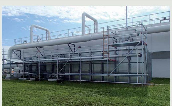
MBR system for wastewater treatment facilities targeted at emerging markets
