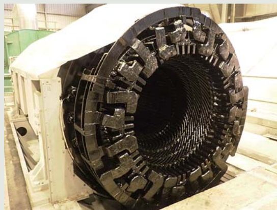
Generator stator rewinding at Joffre Cogeneration Plant, Canada
