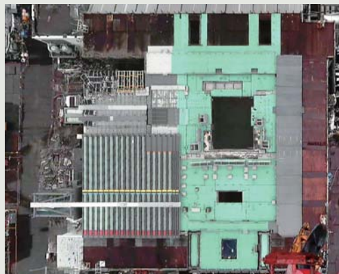
Operating floor of Fukushima Daiichi Nuclear Power Station Unit 3 covered with iron shields in November 2016 (partially not covered)
