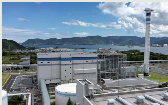
Sakaide Thermal Power Station Unit 2 of Shikoku Electric Power Co., Inc.
