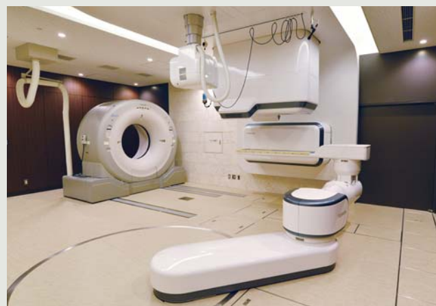
Treatment room of i-ROCK
