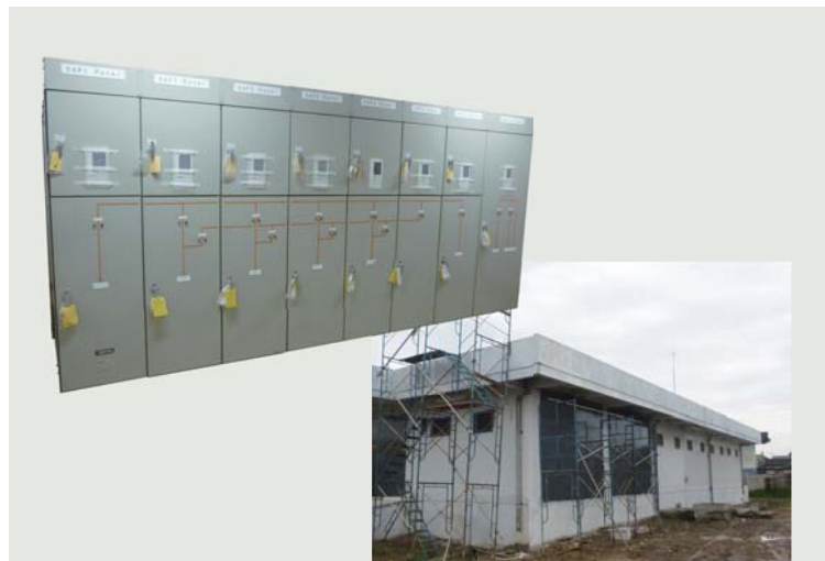
DC switchgear installed at DC feeding substation in conjunction with double double-tracking of Blue Line (Jakarta Kota-Bekasi), Indonesia
