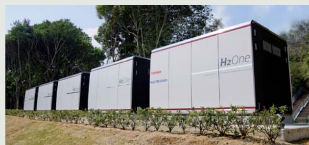
H 2 One™, Toshiba's hydrogen-based autonomous energy supply system, at the Phase 2 building of Henn na Hotel in the Huis Ten Bosch theme park, Nagasaki
