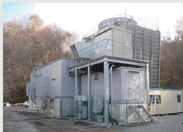
Waita Geothermal Power Plant equipped with skid-mounted wellhead generator
