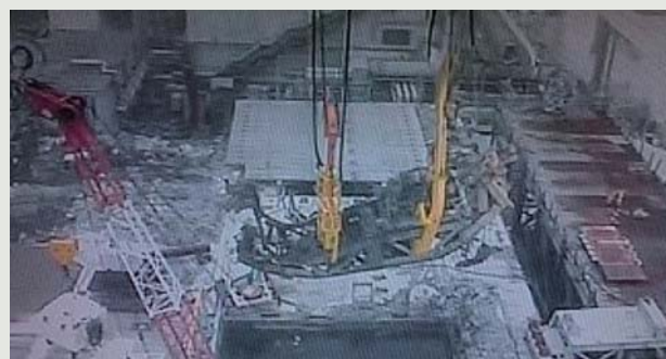
Fuel handling machine removal operation at site
