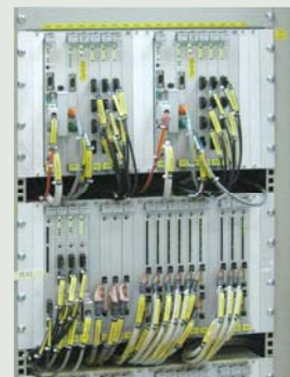
Migration of control system for Tanjung Bin Power Plant Unit 2, Malaysia, using TOSMAP-DS™/LX controllers
