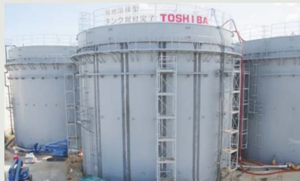
Installation of on-site-assembled tanks
