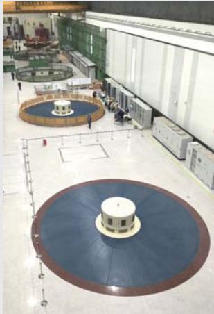
◀ 清遠揚水発電所の全景 Qingyuan Pumped Storage Power Station, China
