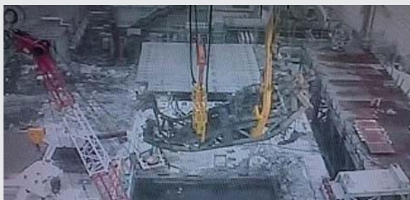
▲ 燃料交換機つり上げ Fuel handling machine removal operation at site
