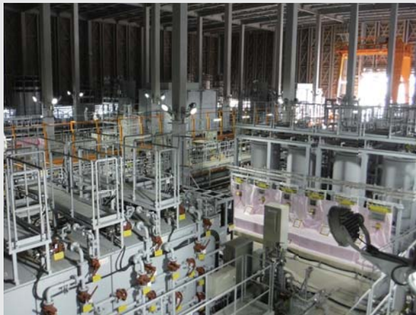
▲ 増設多核種除去設備の全景 Multi-radionuclide removal system at Fukushima Daiichi Nuclear Power Station
