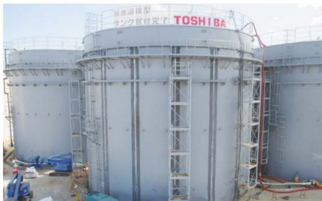
現地溶接型タンクの据付完了 Installation of large-scale on-site-welded tanks
