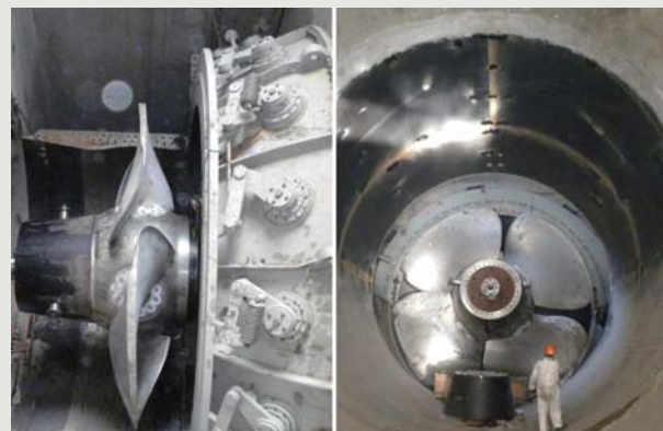
Runner assembly at site of Huangfeng Hydropower Station, China
