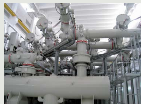
420 kV-80 kA GIS for Al-Zour North "Z" 400/300 kV Substation, Kuwait
