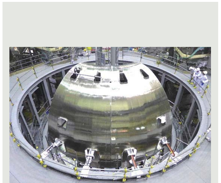
Assembly of two 40-degree sectors of JT-60SA vacuum vessel
