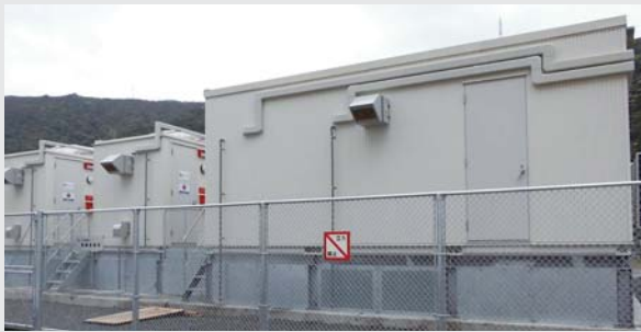
▲ 中種子変電所(上)及び竜郷変電所(下)の蓄電池システム Lithium-ion battery energy storage systems for Naka-Tane and Tatsugo substations of Kyushu Electric Power Co., Inc.
