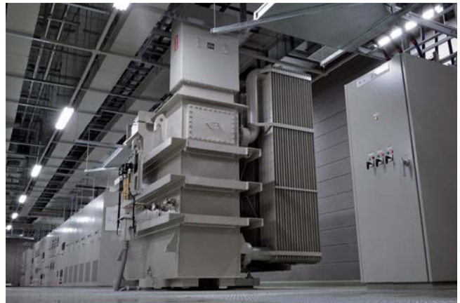
首都高速道路 中央環状品川線 特別高圧受配電設備 Power receiving and distribution system for Central Circular Route Shinagawa Line of Tokyo Metropolitan Expressway
