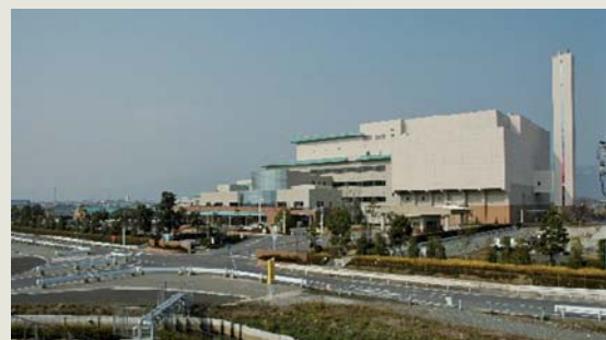
Saga Municipal Waste Incineration Plant
