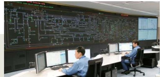
HMI of integrated SCADA system installed in control room
