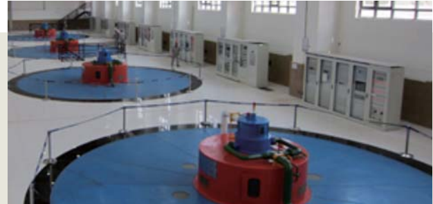
Interior view of Grand Poubara Hydropower Station, Gabon
