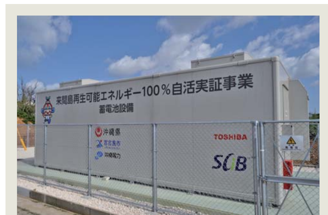
100 kW-176 kWh BESS installed on Kurimajima Island, Miyakojima City, for EMS demonstration project
