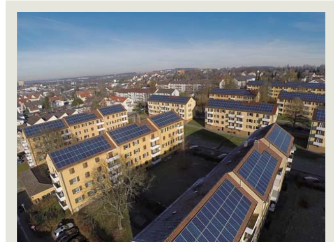
PV system on apartment buildings in Villingen-Schwenningen, Germany
