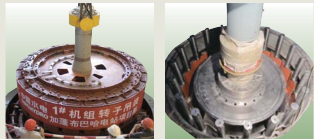
Installation of generator rotor (left) and runner (right)
