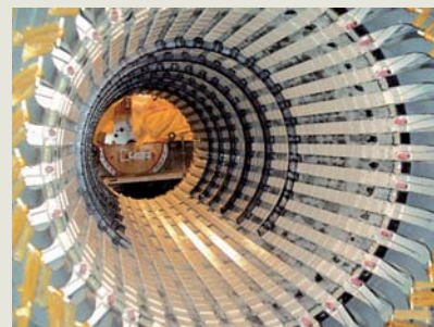
Rewound generator stator for Weston Power Plant Unit 3, U.S.A.
