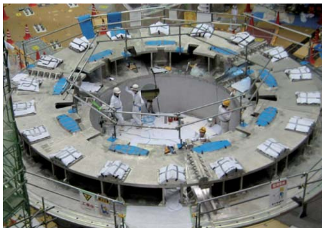
JT-60SA CBの据付け
