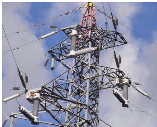
塔上開閉装置 Gas-insulated jumper switchgears (GJSs) for transmission line towers of Hokuriku Electric Power Co., Inc.
