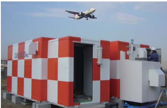
LDA transmitter equipment
