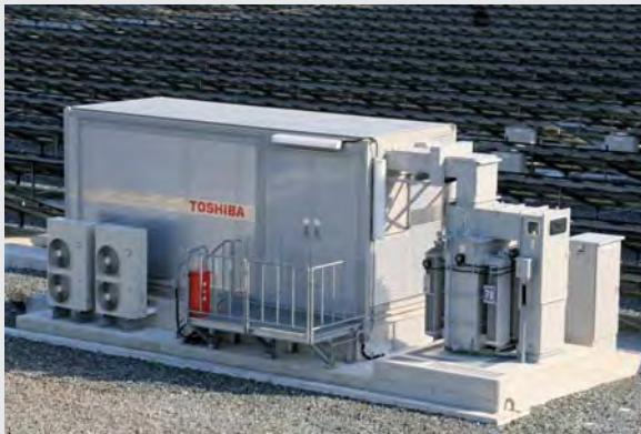
▲ PCSパッケージと昇圧変圧器 Power conditioning system (PCS) package and step-up transformer
