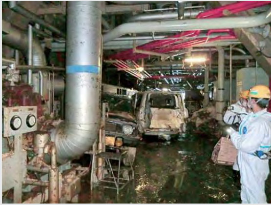
▲ 東京電力(株) 広野火力発電所 震災直後 Hirono Thermal Power Station immediately after Great East Japan Earthquake
