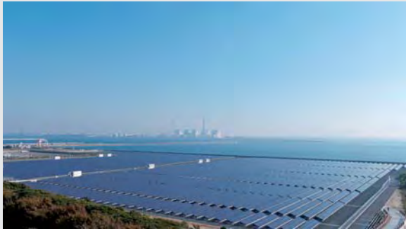
▲ 太陽電池アレイ Photovoltaic (PV) arrays at Mega Solar Taketoyo facility, Taketoyo Thermal Power Station, of Chubu Electric Power Co., Inc.
