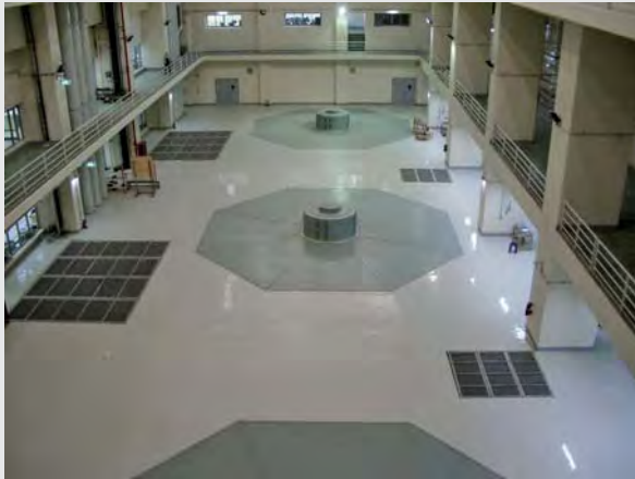
▲ ナムグム2水力発電所の発電機フロア Interior view of Nam Ngum 2 Hydroelectric Power Station, Laos
