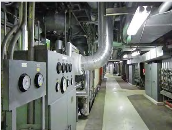
▲ 同 復旧後 Site after restoration of earthquake damage
