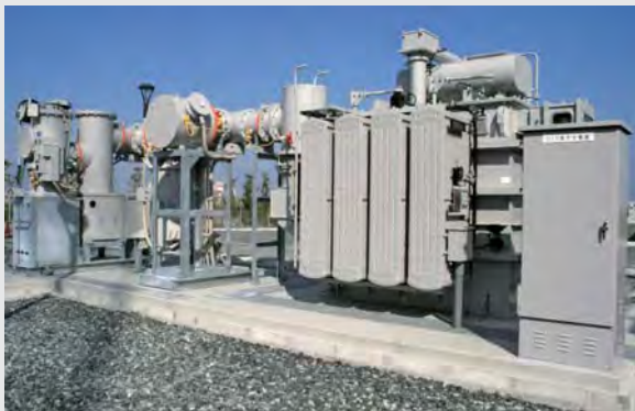
▲ GISと主変圧器 Gas-insulated switchgear (GIS) and main transformer
