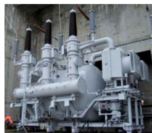
80 MVA-144.5 kV GIT on site after installation
