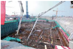
(c) First concrete pouring at Haiyang Unit 2 (June 2010)
