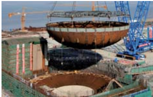
(a) Installation of CV bottom head at Sanmen Unit 1 (December 2009)
