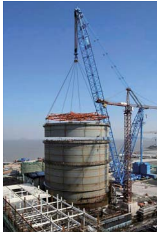
(b) Installation of CV ring #4 at Sanmen Unit 1 (September 2010)
