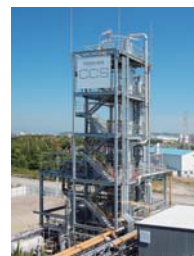
PCC pilot plant at Mikawa Power Station
