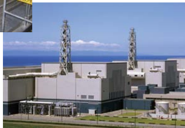
柏崎刈羽原子力発電所と6号機の主蒸気隔離弁の作動確認試験 Kashiwazaki-Kariwa Nuclear Power Station (right) and functional test of main steam isolation valve for Unit 6 (left)
