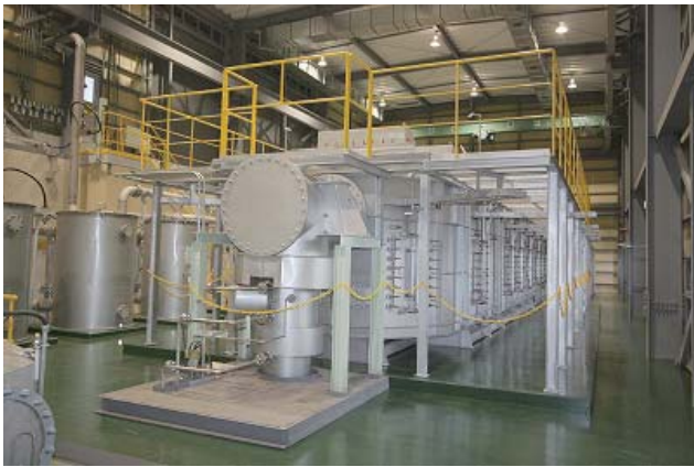
Remediation facility for PCB-contaminated soil
