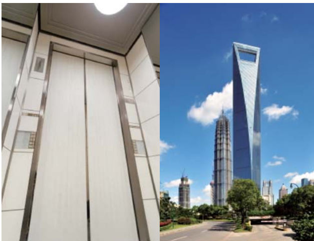
(a) View from inside the car of a super-high-speed elevator
