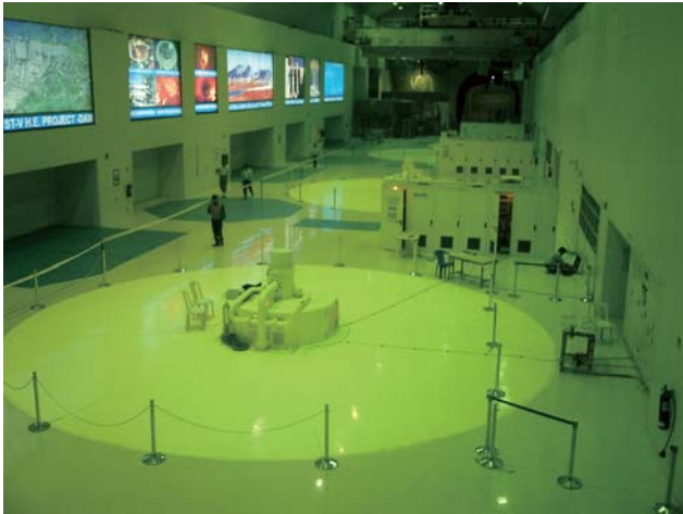
View of Teesta Stage V Power Station
