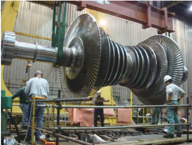
Installation of low-pressure (LP) turbine rotor
