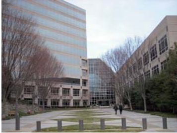
New office of Toshiba America Nuclear Energy (TANE), located just outside Washington DC
