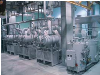
TransGrid Haymarket Substation GIT/GIR
