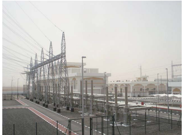
Completed building for 220 kV GIS
