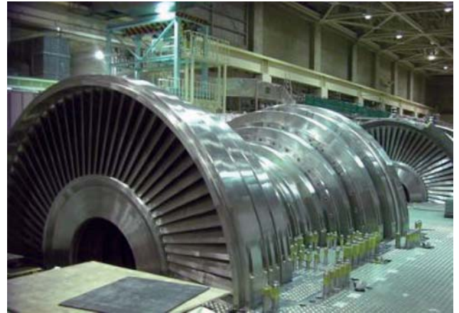
Assembly work for high-efficiency turbine
