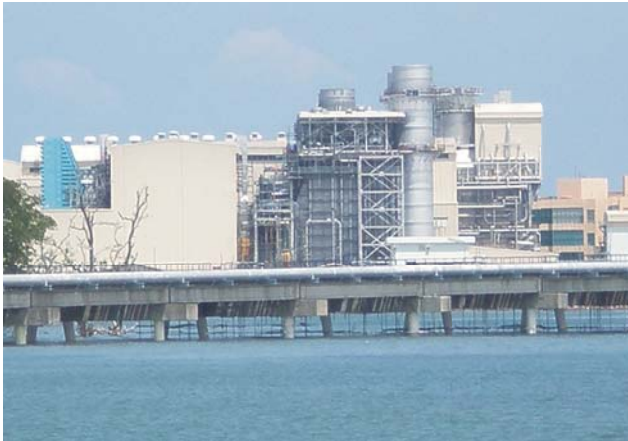
Multishaft combined-cycle power plant for the Port Dickson Rehabilitation Phase 2 Project
