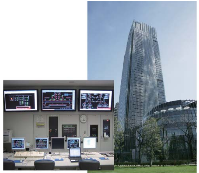
Tokyo Midtown and view of control room
