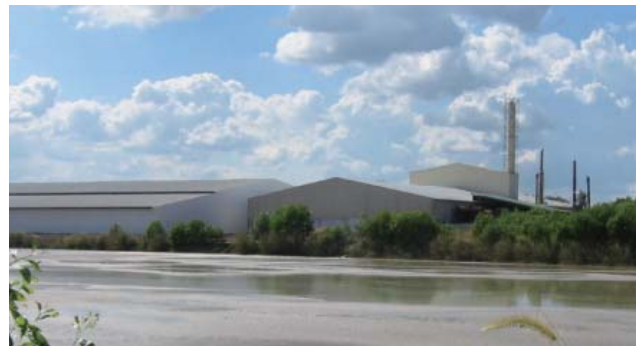
Existing lagoon of tapioca starch processing company
