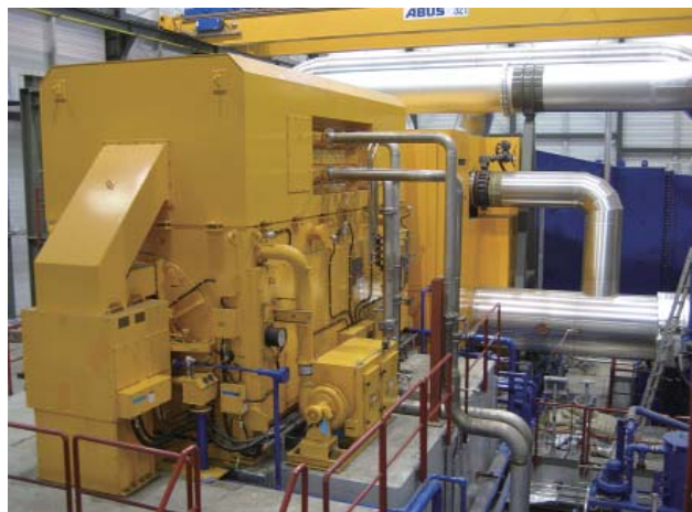
Turbine and generator set for 33.6 MW Low-Pressure Unit of Hellisheidi Geothermal Power Plant, Iceland
