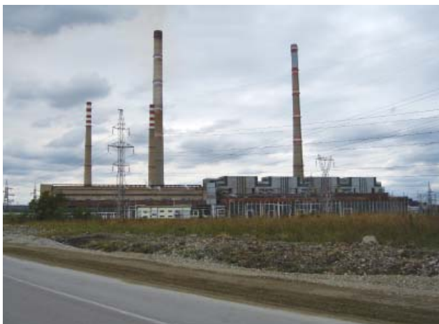
Maritsa East II Coal-Fired Power Plant, Bulgaria
