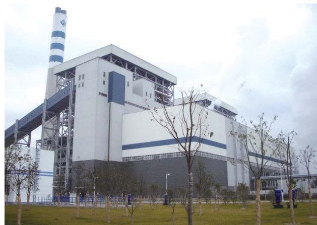
Taizhou Ultra-Supercritical Thermal Power Plant, China
