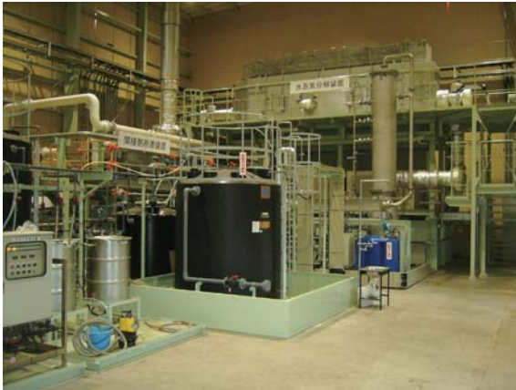
PCB汚染土壌処理施設 Remediation facility for PCB-contaminated soil
