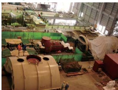
Installation work for power train
