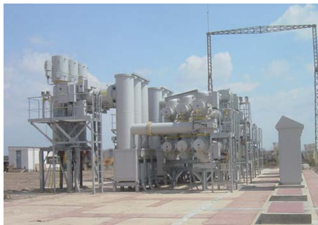
420 kV gas-insulated switchgear (GIS) at Brazi Vest Substation, Romania
