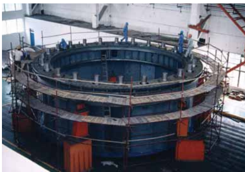
75 MW Kaplan turbine shop assembly at THPC
