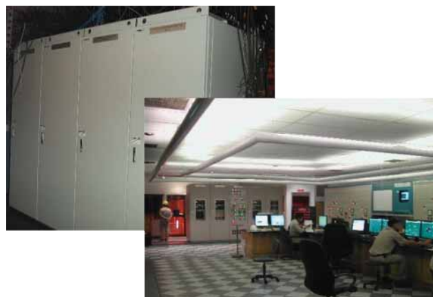
Digital control system for steam turbine and generator
