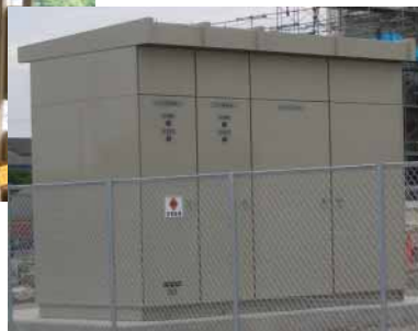
36 kV 固体絶縁スイッチギヤ 36 kV solid-insulated switchgear (SIS)
