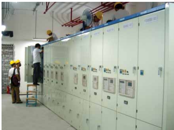
現地で据付け中のC-GIS Installation of cubicle type GIS at site
